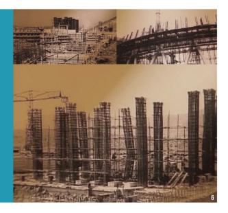
Construction of 59 meters high Otllovici dam was almost finished in October 1979, and a road was bulk along the pipeline from dam to thermal power plant. Works on 250m high TPP chimney were completed on June 8th, 1979. Approximately 80 employees were engoged and they embedded 3,100 m3 of concrete and 800 tons of reinforcement bors.
