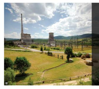
Being a responsible business company, Elektroprivreda Crne Gore strives to stablish an optimal synergy level between its energy facilities and environment. We improved de-dusting system of TPP Pjevlja by assembly of a contemporary electrostatic precipitators in 2009, and thereby reduced particles emission from the average 350 mg/l/m3 to 15 mg/l/m3.
